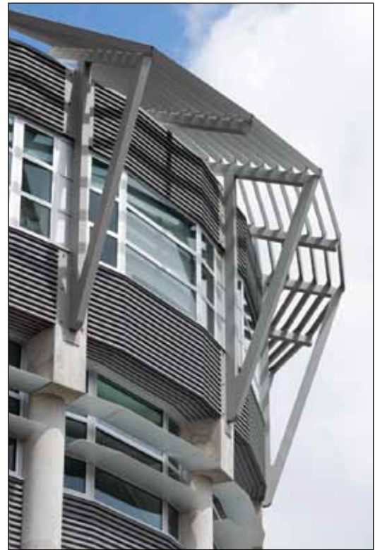
Figure 1 Windows on top floor feature sunshading devices
